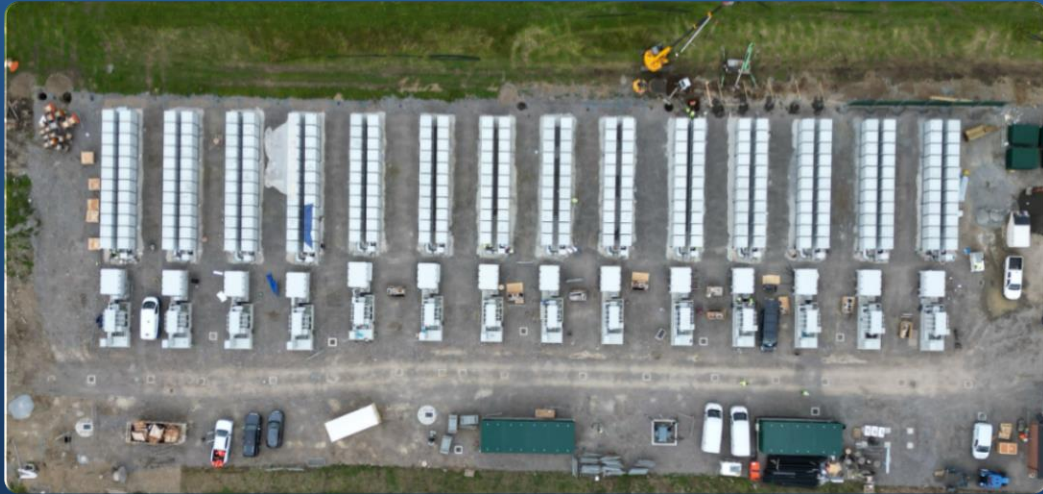
📍 The UK Auchteraw Independent Energy Storage Power Station Project
